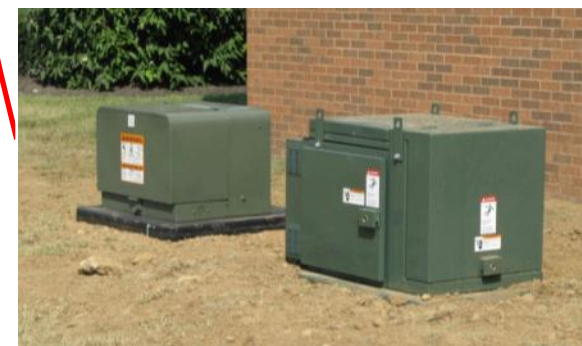
Storage Close to Customer 25-50 kW
